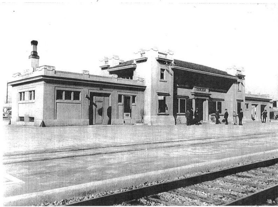
Gilroy's New Train Depot 1918
